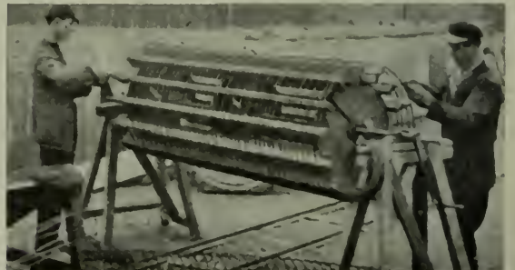
FIG. 6. TYING ANNULAR REINFORCEMENT TO LONGITUDINAL BARS.
